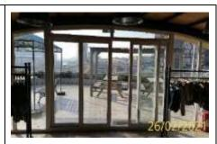
NC-6: Showroom emergency exit is sliding glass door, which is not complaint with the local regulations.
